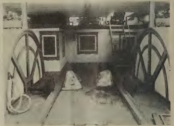
The engine room of the house boat. When the motor car is run in on the skids and its driving mechanism connected the boat is ready to get under way
